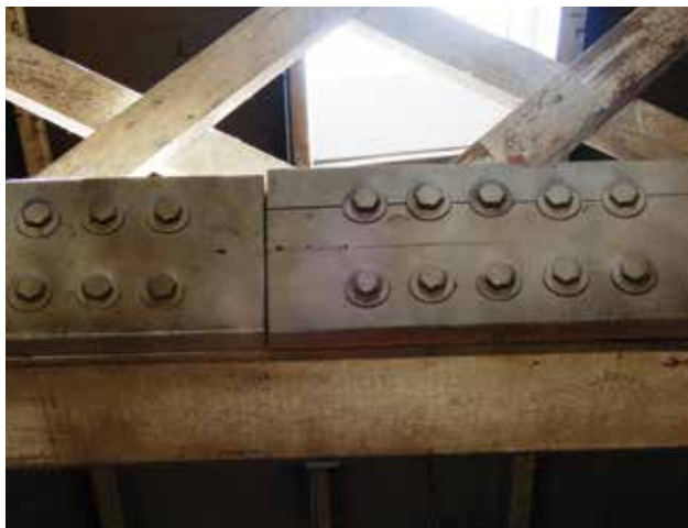
Figure 5. Partial view of lattice truss within the roof structure above the administration building.
