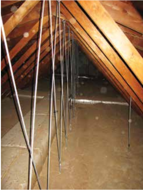
Figure 3. Steel cable reinforcing introduced at roof trusses from Indiana community center.
