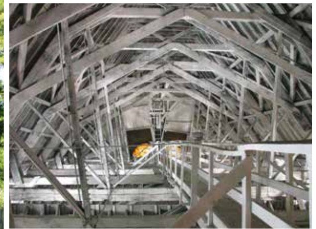
Figure 2. Attic framing from 1860s church in Chicago, Illinois.
