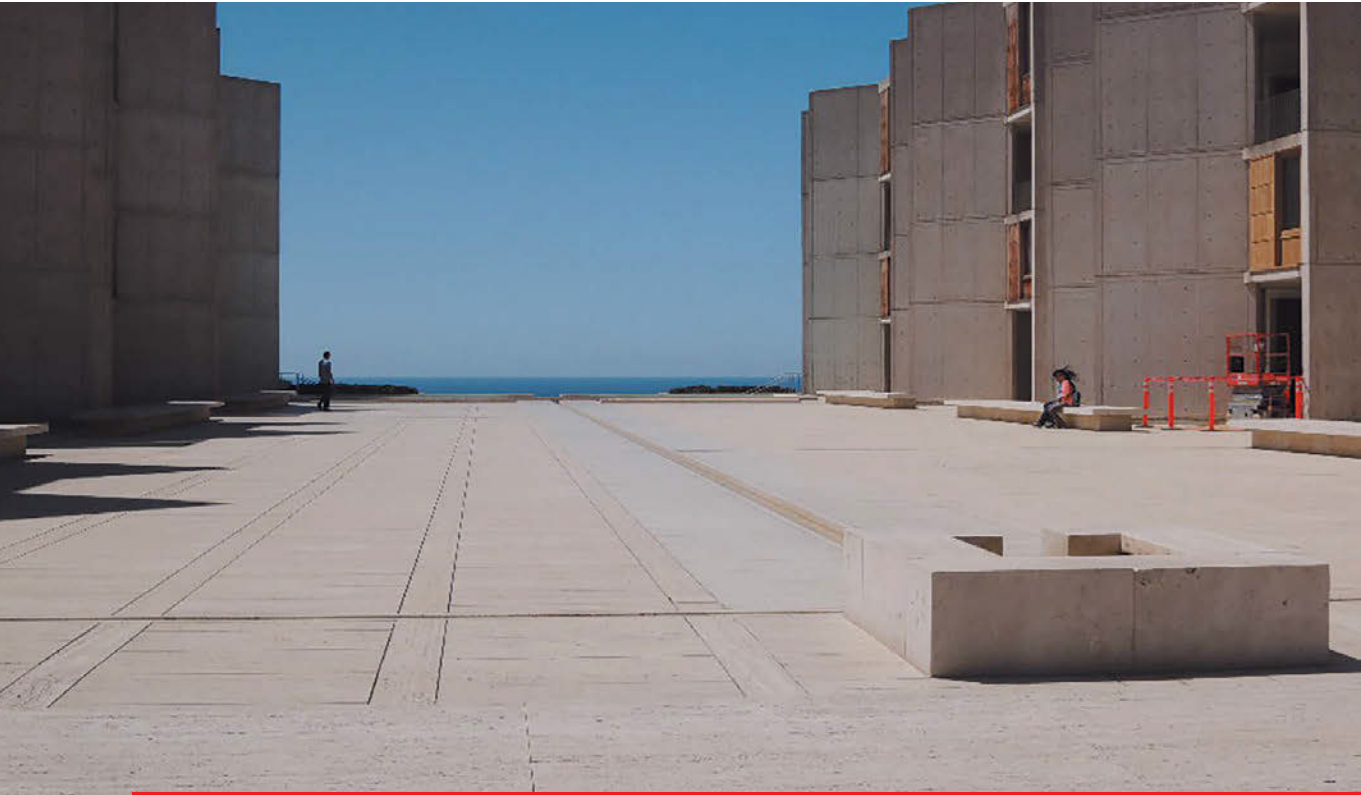
View of plaza looking west (WJE Photo).
