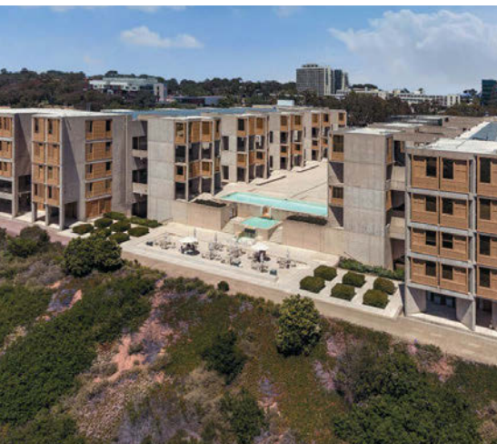
West elevation prior to conservation project (WJE Photo).
