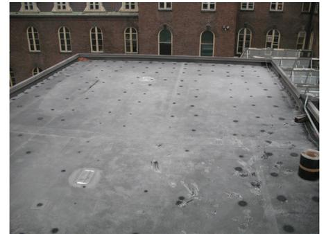
The dark round circles in this photo indicated the insulation's fastener pattern. The fastener plates are frost-free due to thermal bridging. It is estimated that thermal bridging of fasteners reduces the R-value of insulation by eight to ten percent.
