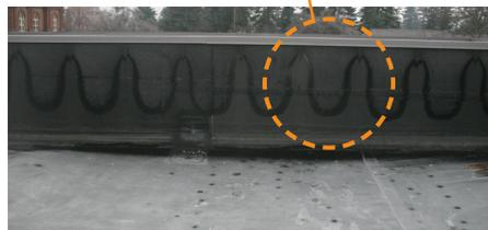
Frost patterns on the EPDM clad parapet walls formed a perfect sine wave. The distance between the peaks of the nonfrosted areas matched the width of the insulated metal wall panels exactly, confirming our earlier observation of air movement from the interior into the roof system, but also vividly showing the degree of heat loss through the joints between panels.
