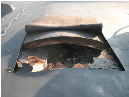
Single layer of polyisocyanurate insulation. The insulation warped as a result of condensation on its underside and fastener corrosion. The source of the moisture was interior air.
