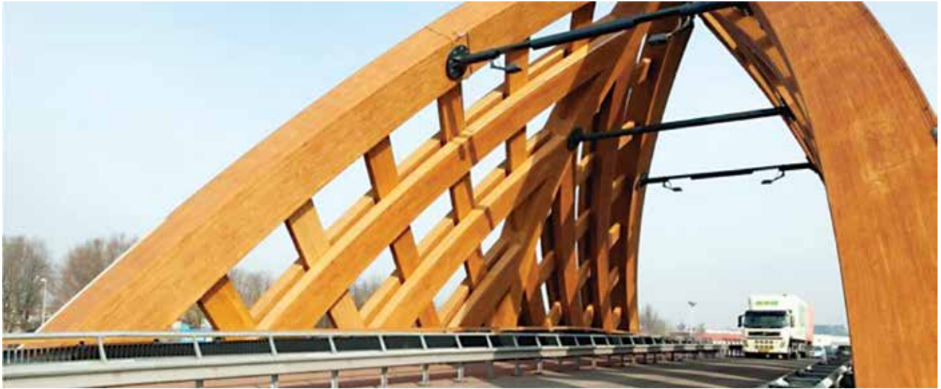
Figure 8. Wood bridge constructed with acetylated Accoya in Sneek, Netherlands Built: 2008-2010. (Photo Courtesy of Accsys)
