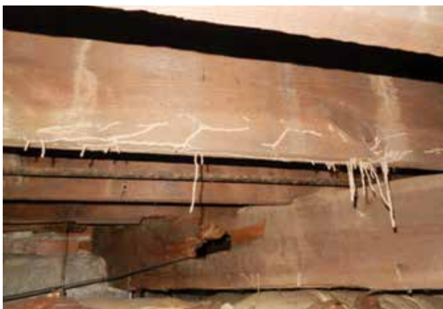
Figure 3. At lower moisture contents certain wood species are vulnerable to insects. (Crowe Photo)
