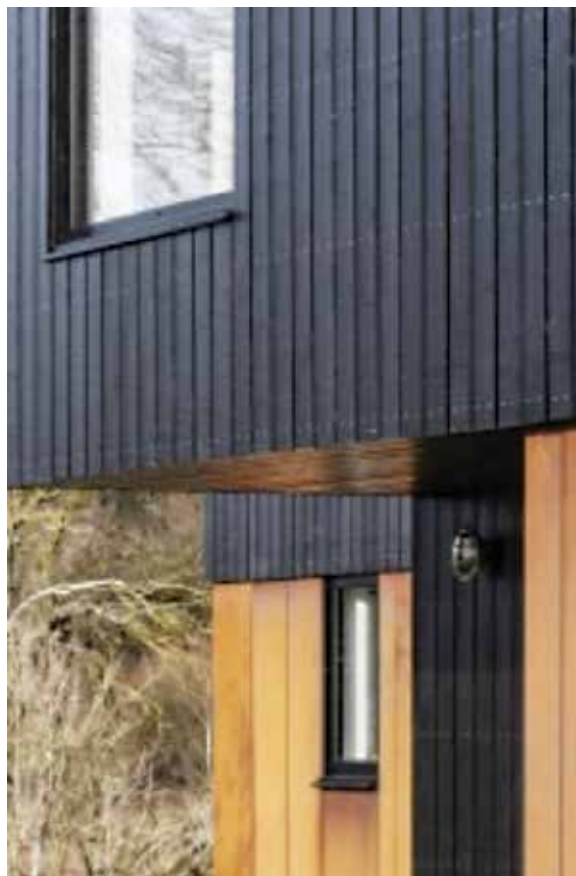
Figure 6 Image of Russwood Thermopine®, design by Fife Architects, photo by Keith Hunter.
