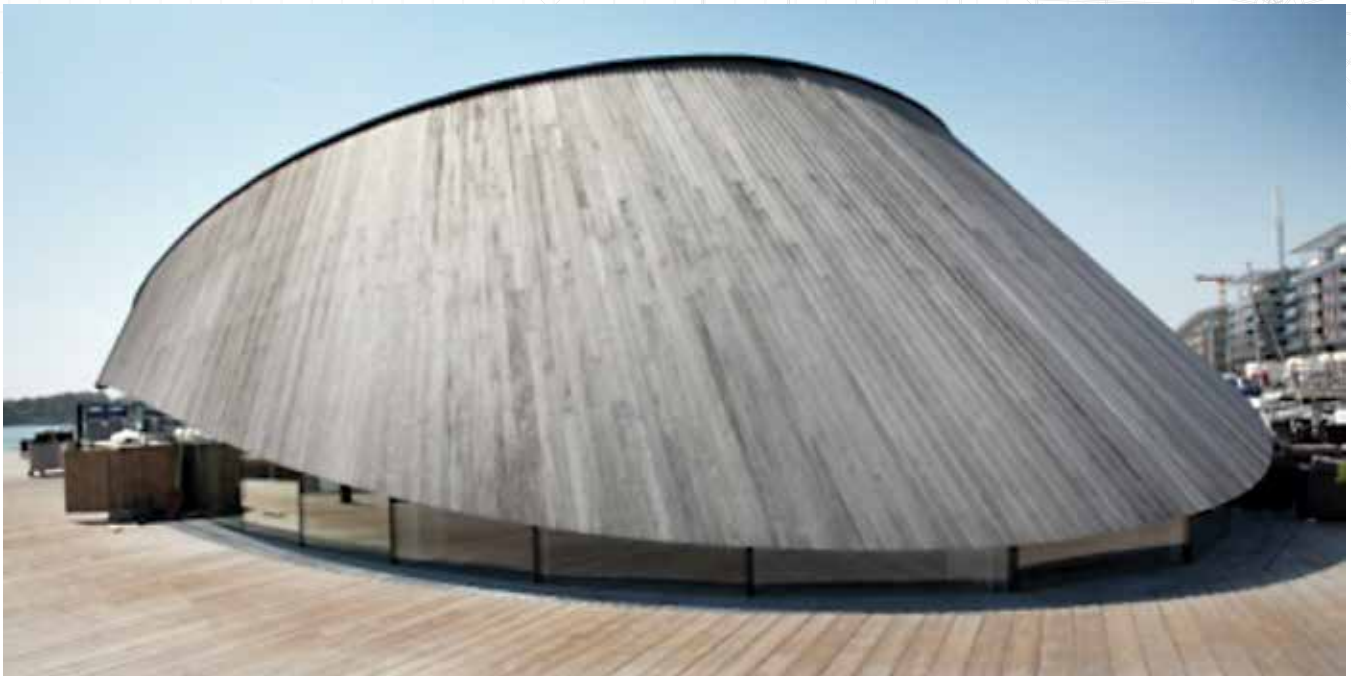
Figure 7. Photo courtesy of Kebony shows Kebonized wood cladding and decking (SYP) at Onda Restaurant in Oslo, Norway.
