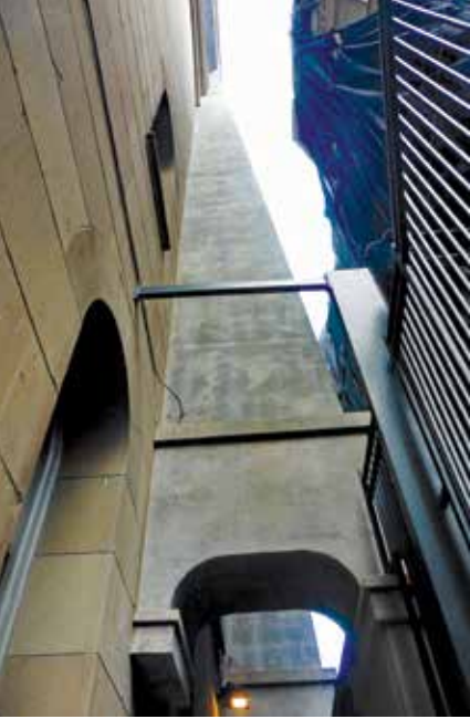
Figure 5. Pilaster end supported on rocking block in north alley. Courtesy of Charley Stern.
