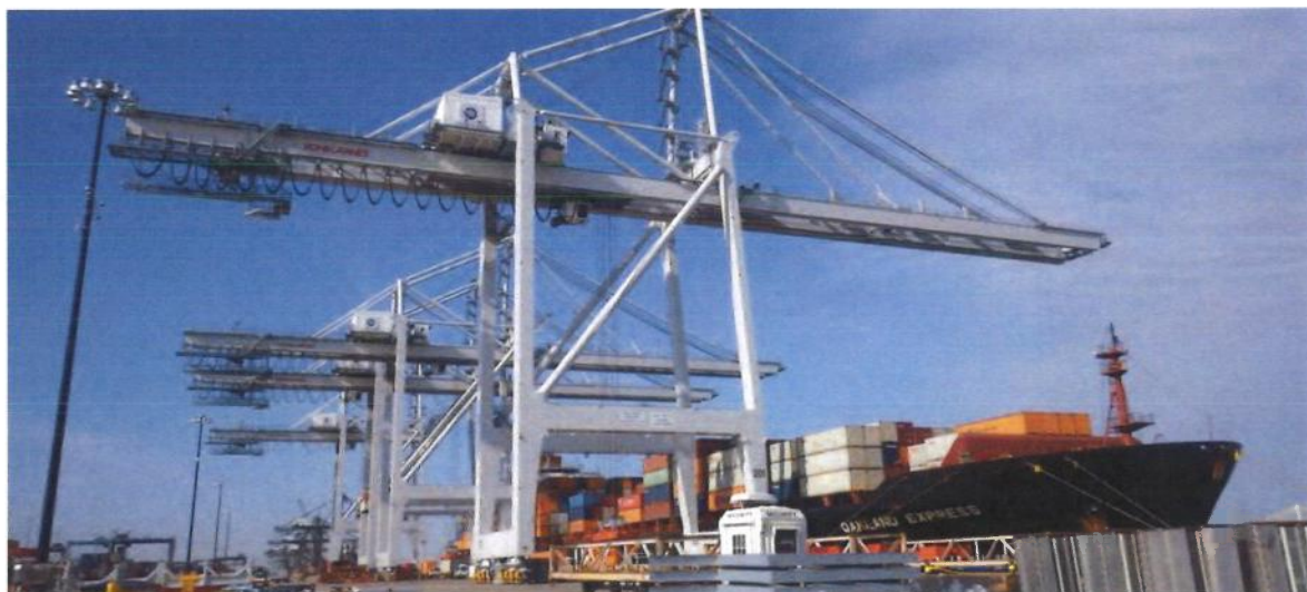
Figure 1—New STS container cranes at BCT.
