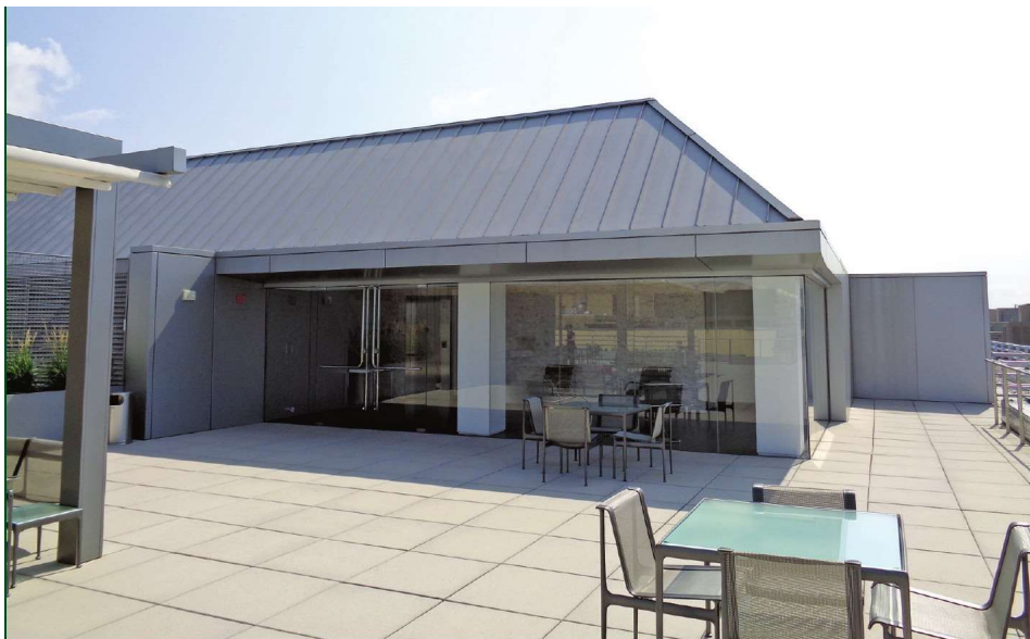
Figure 7. New interior conditioned spaces must be properly integrated into the existing primary building enclosure.
