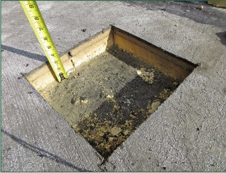
Figure 1. Core cuts or larger destructive openings into the existing roof assembly can be used to confirm components and condition of the in-service roof system as well as results of non-destructive testing. This information will help the design team and owners define necessary repair or replacement scope criteria early on in a project.
