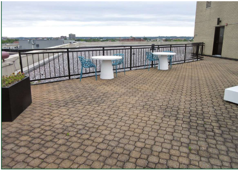
Figure 6. Pavers come in all shapes, sizes, and materials, and they are a common choice for use as walking surfaces at rooftop amenity spaces.
