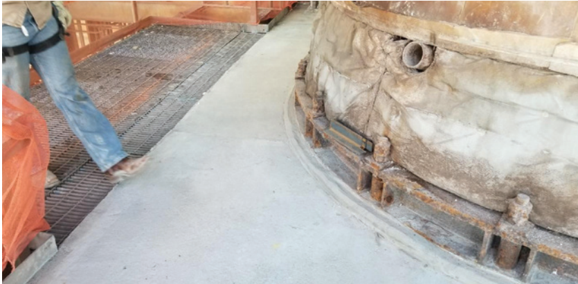
Figure 9. Completed repair on top of upper deck.
