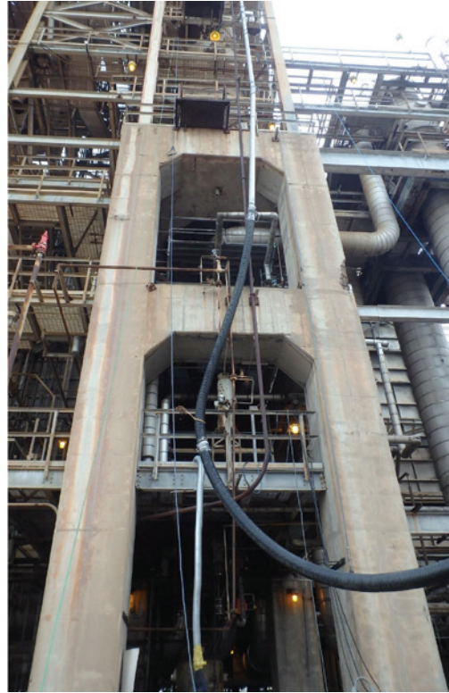
Figure 1. Catalytic reformer support structure.
