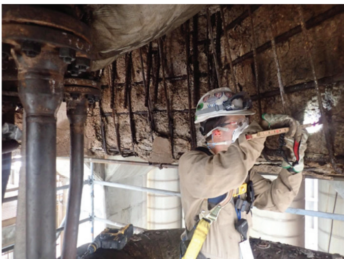
Figure 5. Measuring depth of drilled hole used for chloride and carbonation testing.
